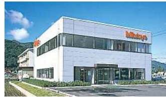
Suwa Sales Office
